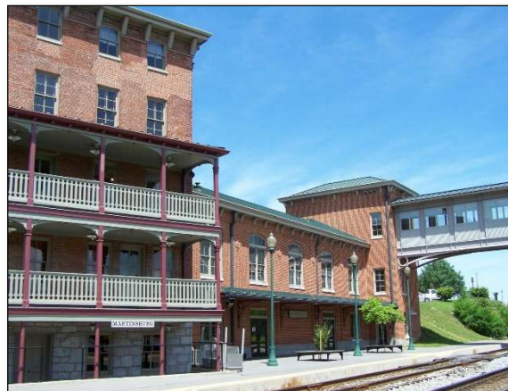
Caperton Station – station corridor to be upgraded.
