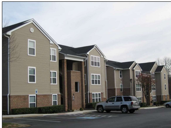
Martins Landing apartment community – Tavern Road.
