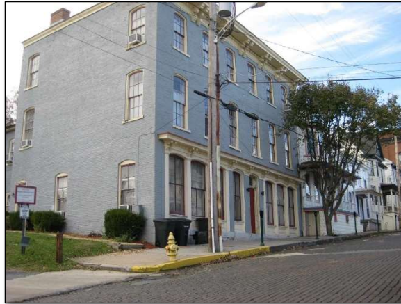
Future streetscape corridor - East Martin Street.
