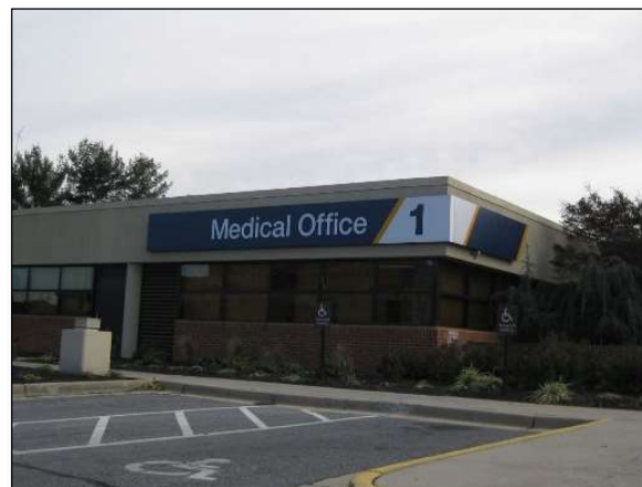
Medical offices supporting Berkeley Medical Center.
