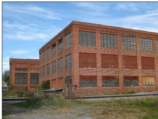
Interwoven Mills – prime for redevelopment.
