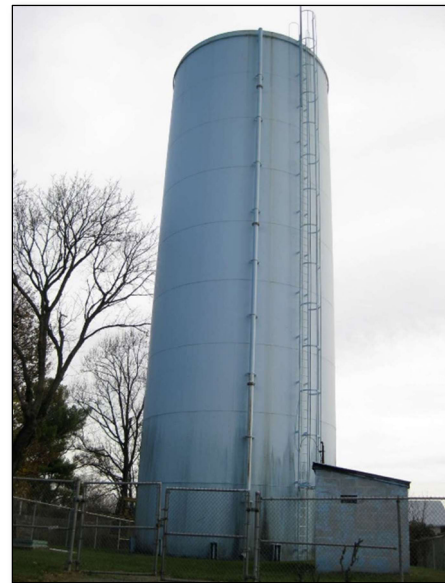
Public water storage – Western Avenue.
