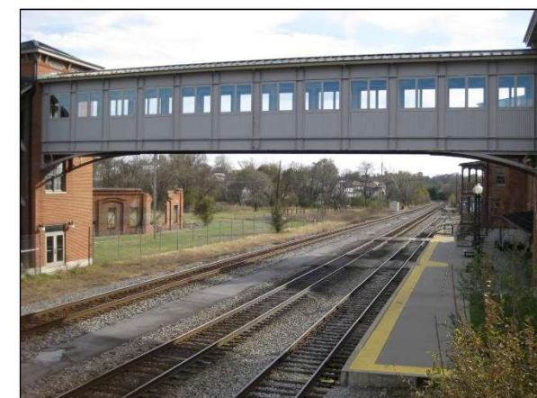
Pedestrian bridge at Caperton Station.
