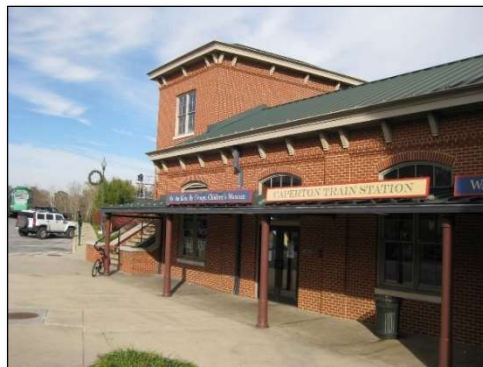
Caperton Station – improvements planned.
