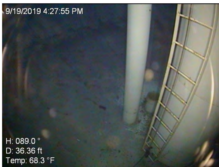
74) The wet interior ladder is in good condition.
