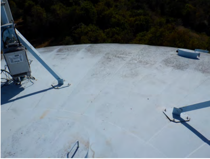
16) The roof coating is in fair condition.
