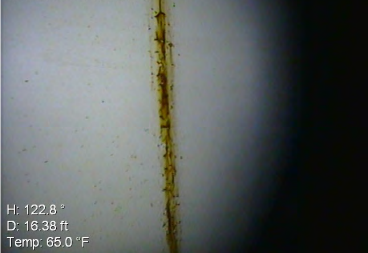
60) Spot coating failures to the substrate on the sidewall.
