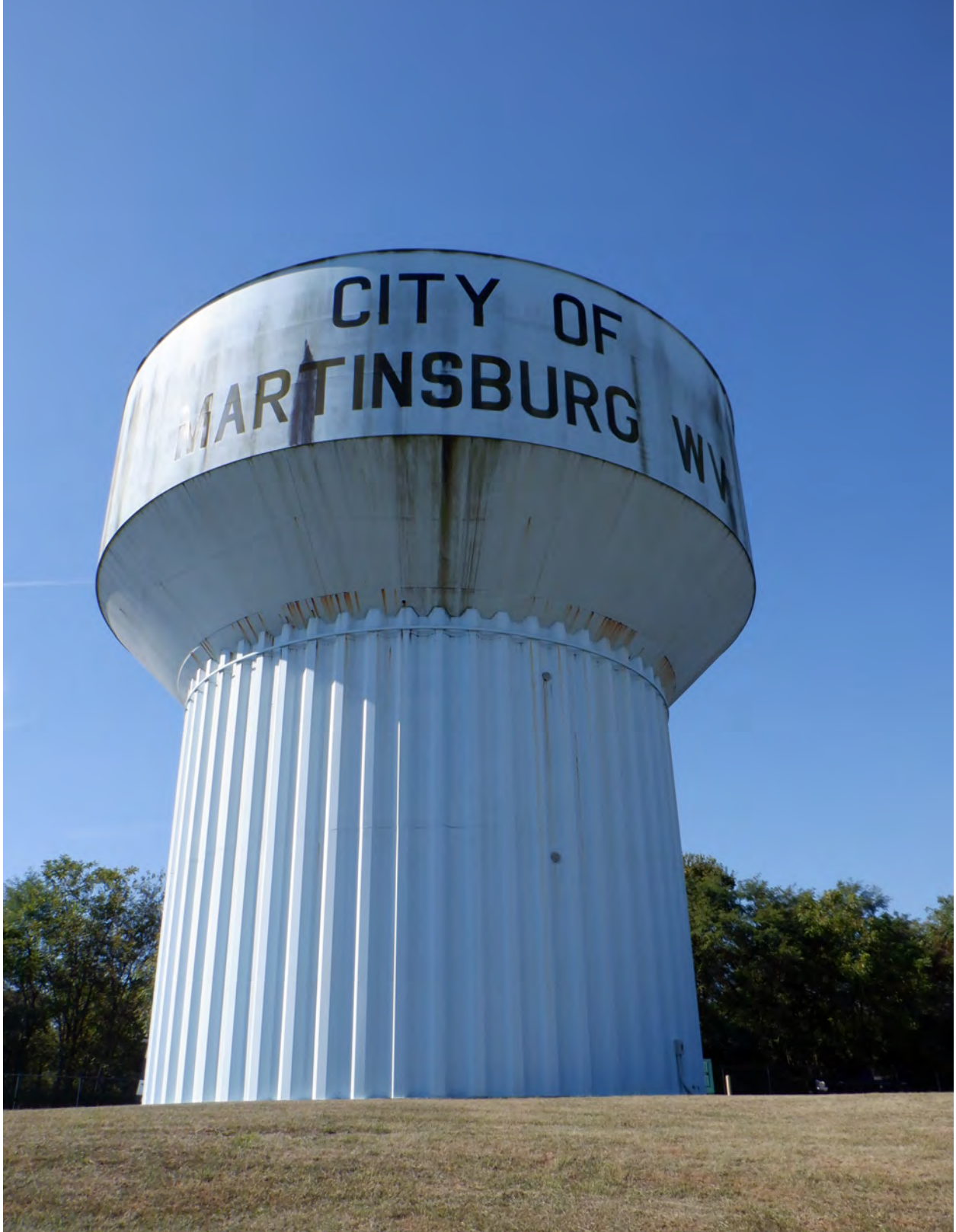
1,500,000 gallon fluted column (Boyd Orchard) owned by the City of Martinsburg, West Virginia.
