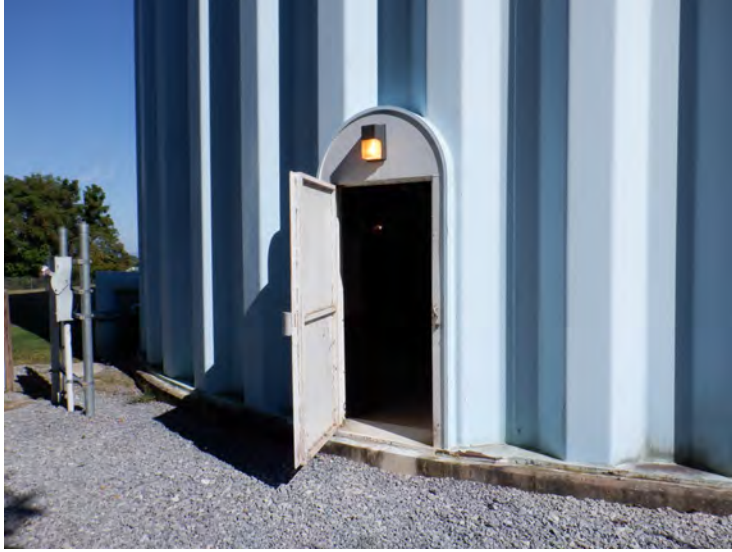
7) The service door was properly locked upon arrival.
