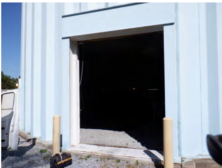
6) The overhead door is in good condition.
