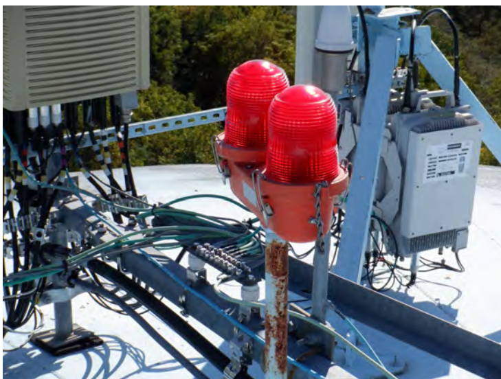
21) The double red aviation light is attached to a free standing pole.
