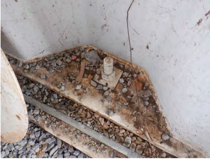
28) The anchor bolts are in good condition.
