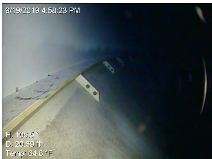
63) The stiffener at the transition is in good condition.
