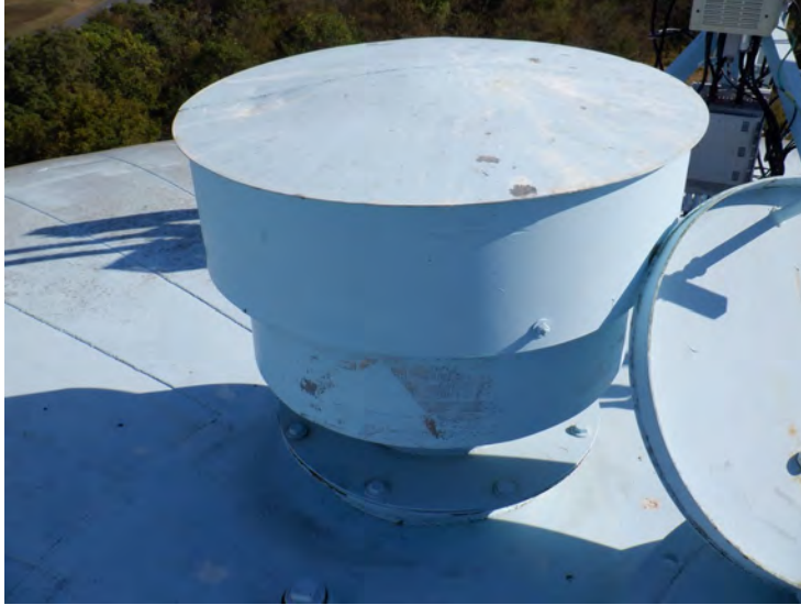
22) The roof vent coating is in fair condition.
