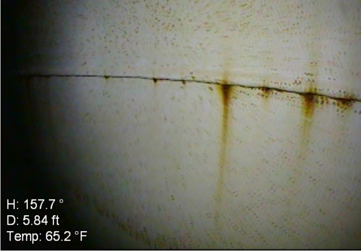
58) Spot coating failures to the substrate on a wet interior sidewall weld seam.
