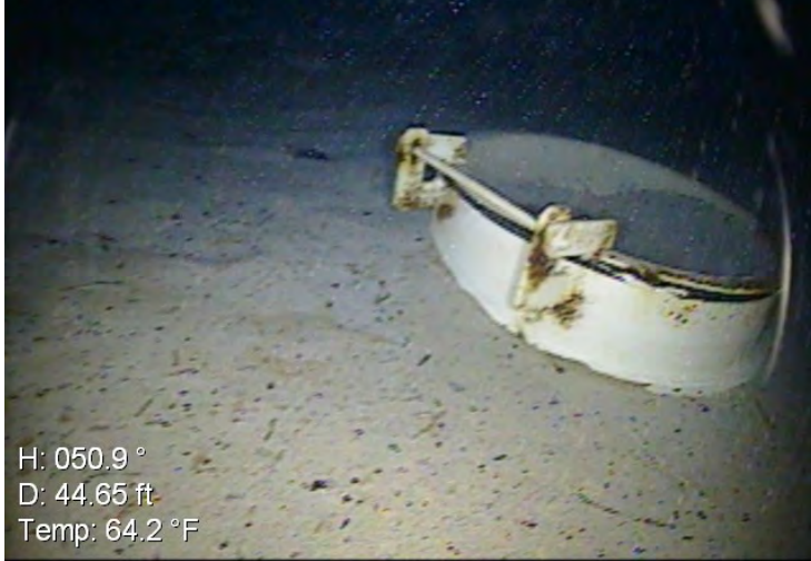
79) The coating on the wet interior manway is in poor condition.
