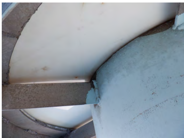
24) The pressure plate on the vent is free to move without interference.
