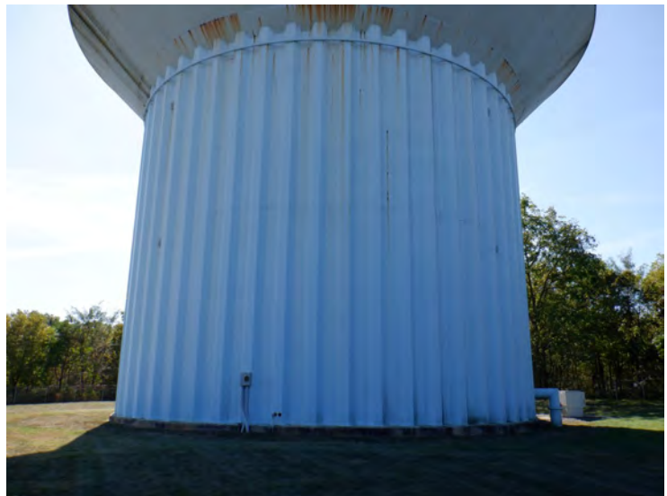
8) The column coating is in fair condition.
