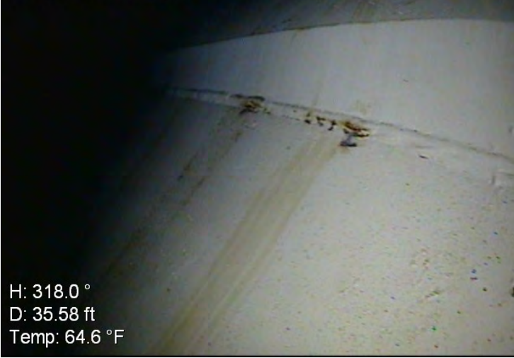
85) Spot coating failures an the upper bowl weld seam
