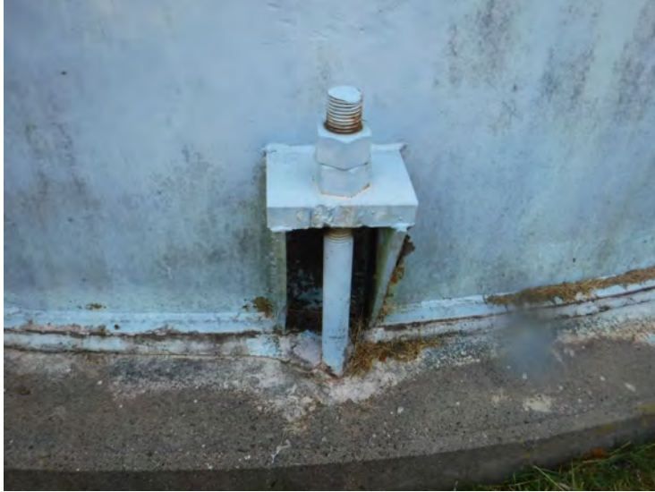
4) Typical anchor bolt is in good condition.
