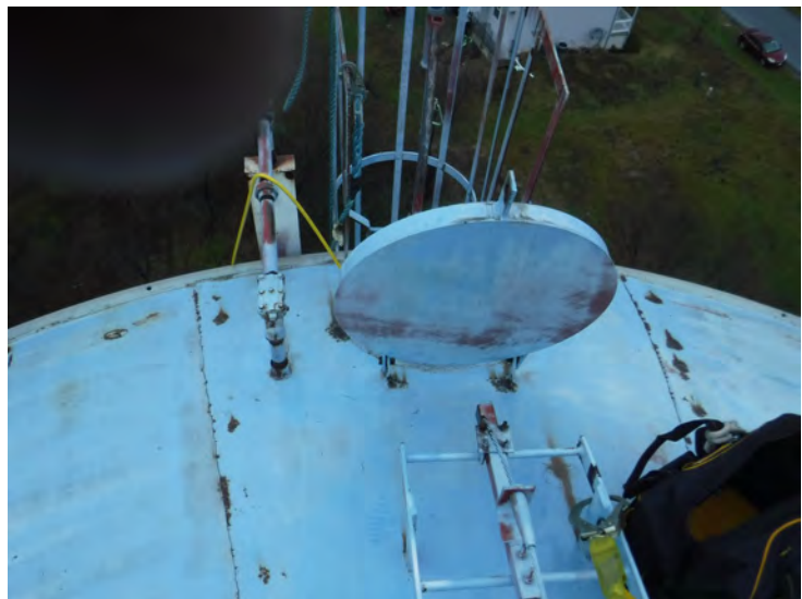
14) The primary roof hatch is in good condition.
