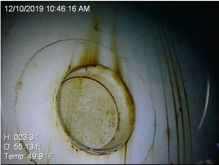
29) The manway penetration is in good condition with rust streaking.
