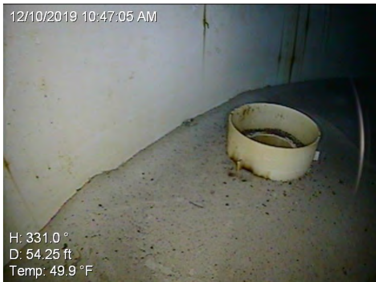
31) The draw pipe is in good condition.
