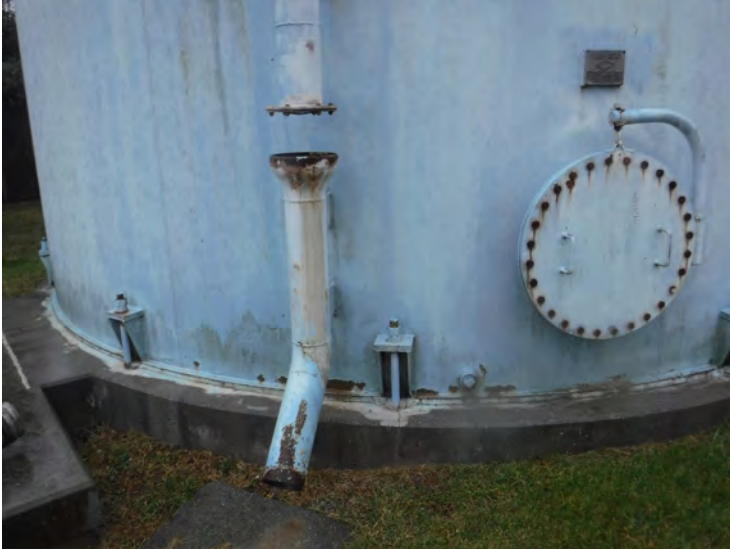
7) The overflow pipe discharge is in good condition.
