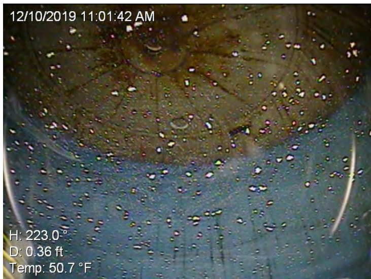
22) The roof viewed from the ROV.
