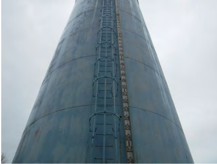
10) The sidewall ladder is in good condition.
