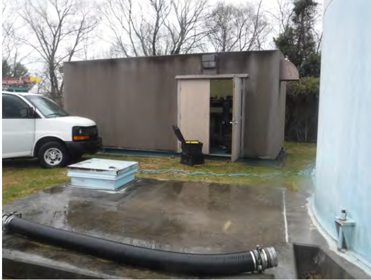
34) There is piping located in a building next to the tank.
