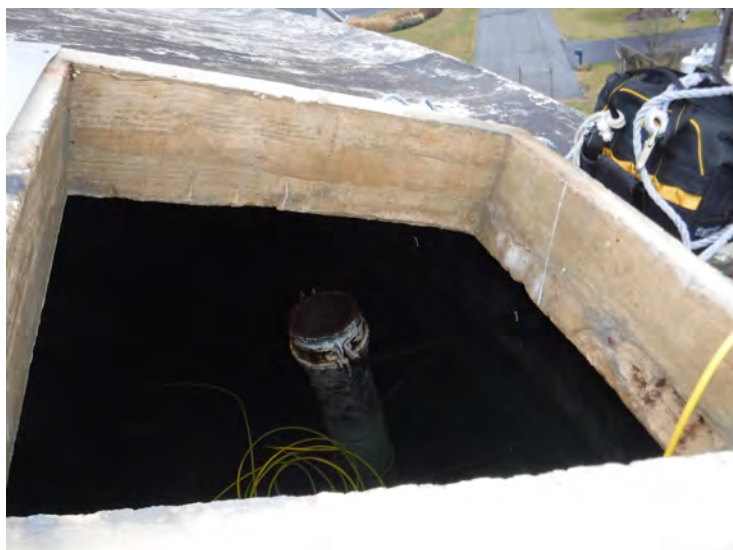
12) The concrete roof hatch curb is in good condition.
