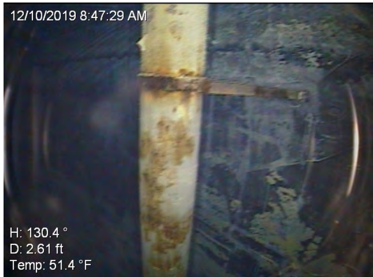
17) The overflow pipe coating is in fair condition.
