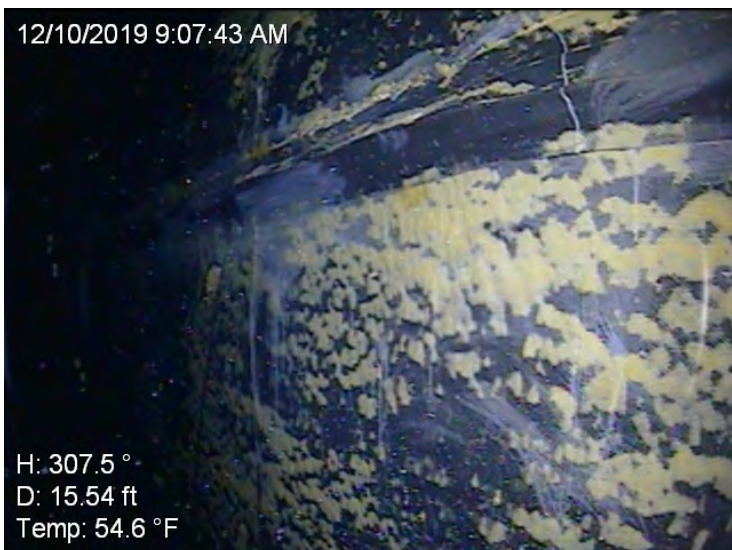
18) The rubber membrane on the sidewall is in good condition.
