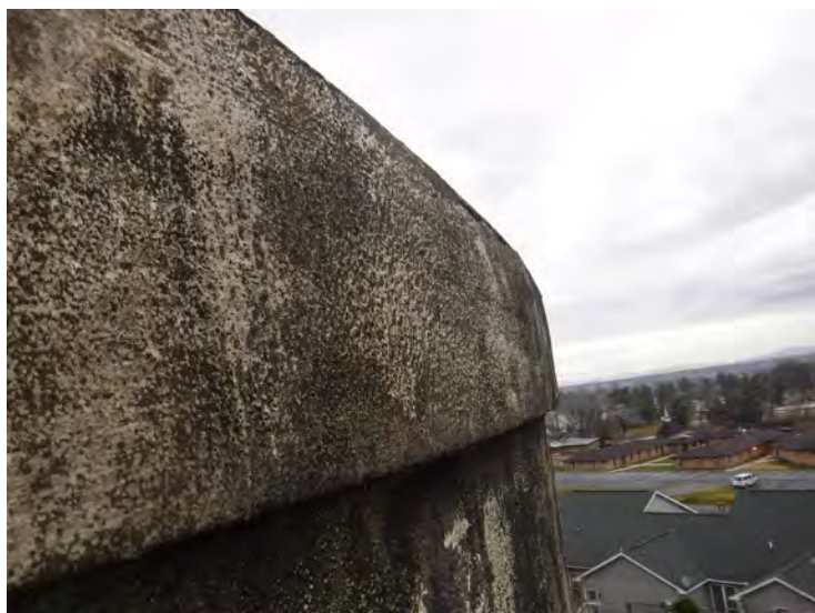
6) The tension ring at the top of the sidewall is in good condition.
