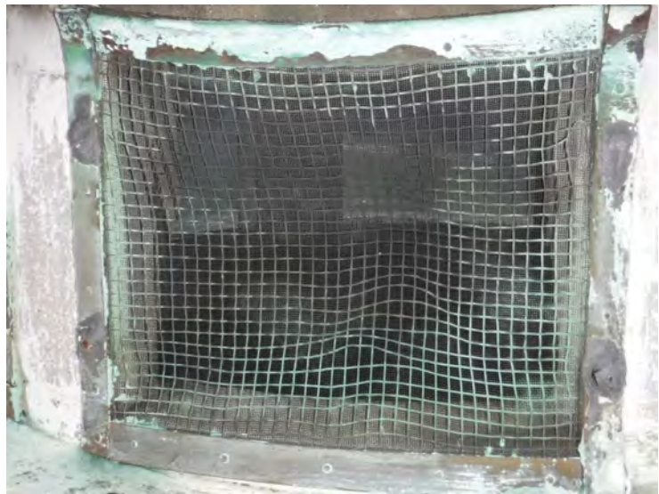
11) The vent screens are in fair condition.
