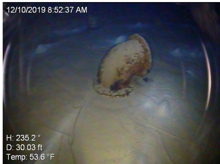
20) The fill/draw pipe is in good condition.
