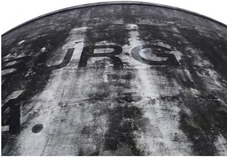
4) The sidewall coating is in poor condition.
