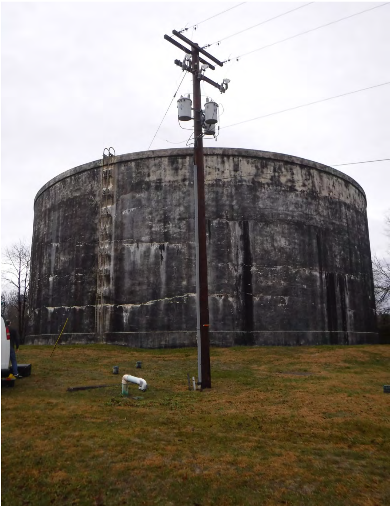
2,000,000 gallon reservoir owned by the City of Martinsburg, West Virginia.
