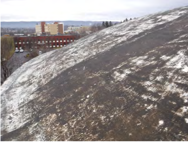
7) The roof concrete is in good condition overall.
