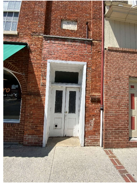
Queen Street Stair Entrance
