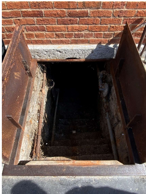
Partial Basement Sidewalk Access
