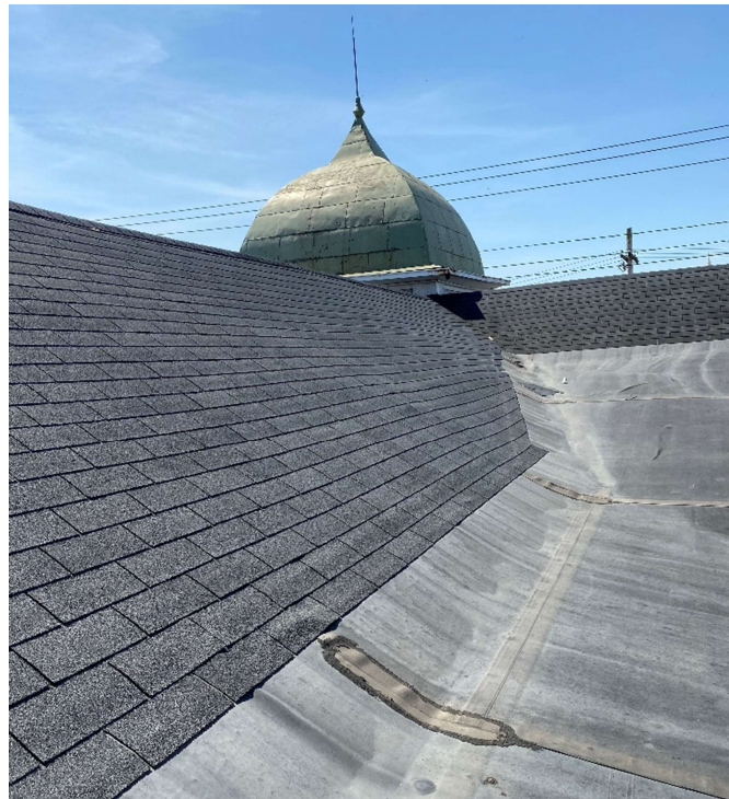
Asphalt Shingles and Rubber Membrane
