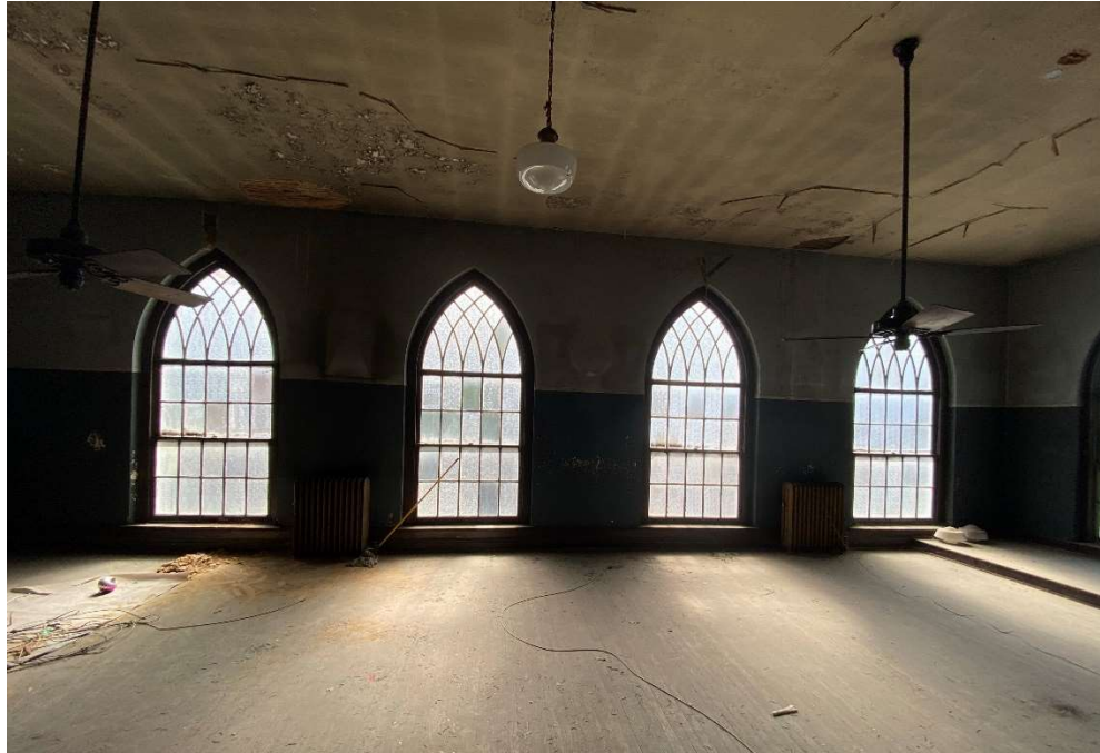
East End Ballroom window wall facing Queen Street
