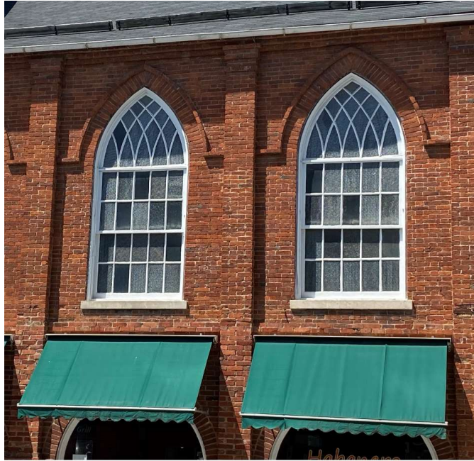
Queen Street Elevation Pointed Arched Windows and Solar Controls
