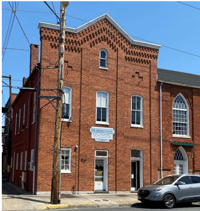
Burke Street Elevation Windows
