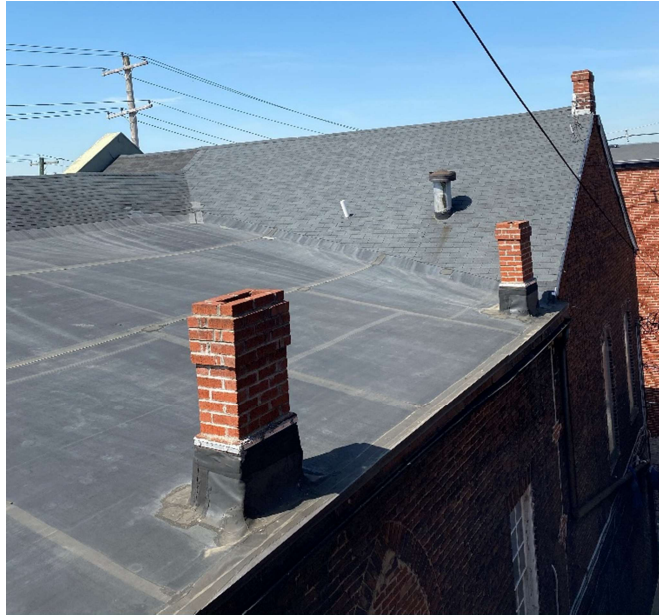
Rubber Membrane Roofing and Chimney Flashing
